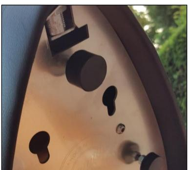
**Step 13:** Set the new coverplate in place and screw in the four original rubber buffers. Adjust the height of the buffers so they evenly lie on the tank when the seat is closed.
