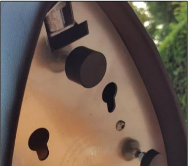
**Step 13:** Set the new coverplate in place and screw in the four original rubber buffers. Adjust the height of the buffers so they evenly lie on the tank when the seat is closed.
